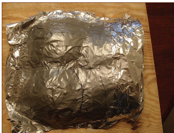
FIGURE 3-43: A single layer of duct tape laid over the foil with minimum overlap
