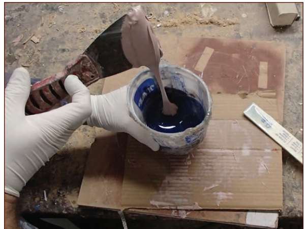
FIGURE 2-40: Blob of Bondo blobbed into mixing cup of resin to make a superblob
