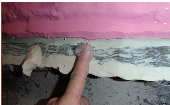
FIGURE 7-49: Applying petroleum jelly as a release agent. Icky.
