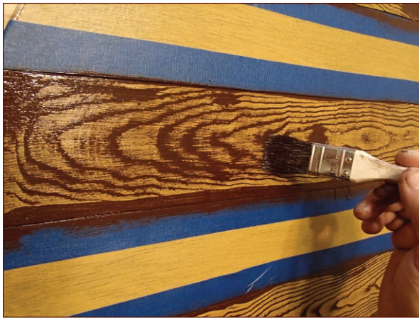
FIGURE 12-20: Dragging some of the stain with a bristle brush to soften the high contrast of the wood grain.
