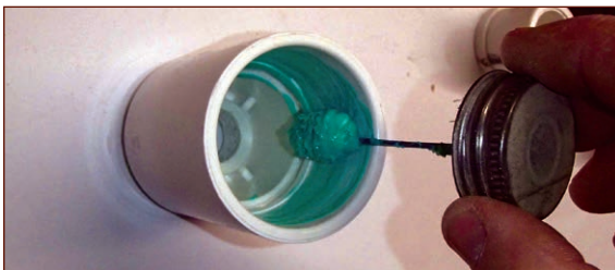
FIGURE 1-76: Apply glue on the inside, not the outside
