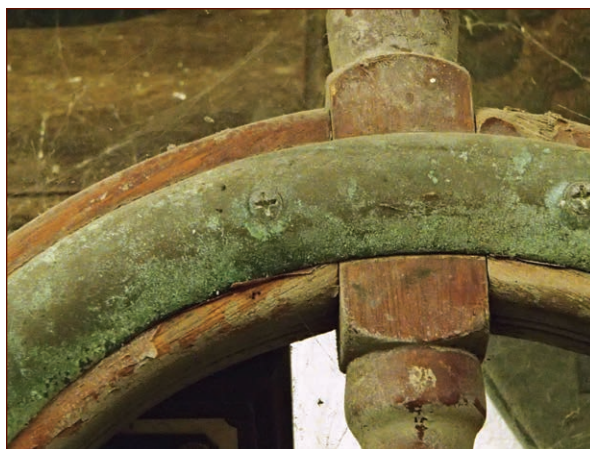
FIGURE 13-42: A strip of bronze after years in a marine environment
